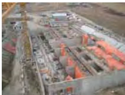
Bearspaw WTP, Calgary, AB - a DBB project - under construction
